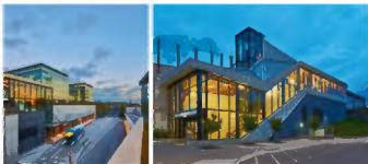
6 Mississauga Transitway MiWay Stations Eight Stations: Cawthra, Central Parkway, Dixie, Etobicoke Creek, Orbitor, Spectrum, Tahoe and Tomken
