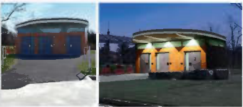
3 Fallingbrook Community Park Washroom 5135 Fallingbrook Drive, Ward 6
